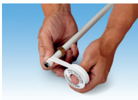
Apply PTFE tape if required
