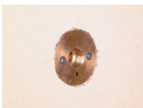
Fig. 48 Installation of HX102W terminal fitting plate and HX101/15W, 15mm conduit terminal
