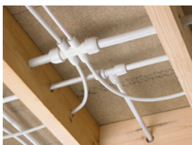
Fig. 29 Hep 2 O speeds up installations because pipework can be easily cabled through drilled joists
